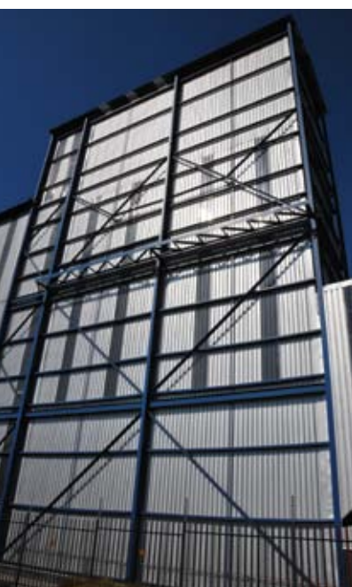
The new 35 metre high processing tower
