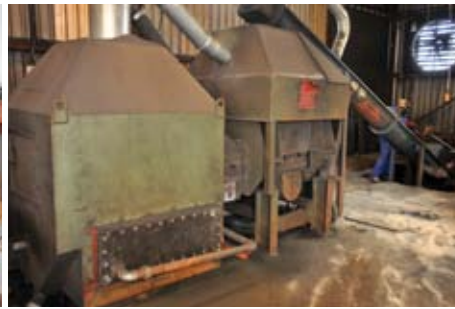
GPM runs on a furane resin based sand system. The foundry also reclaims most of its sand
