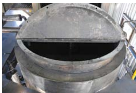
New mixing tanks were installed
