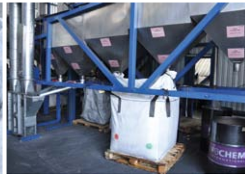
The new screening, sieving and bagging area
